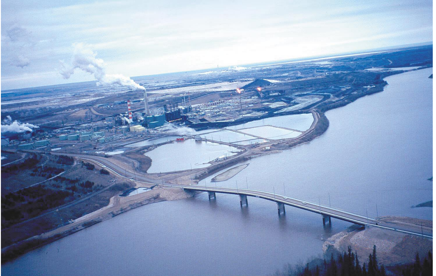
Suncor Energy's oil sands mining operation located north of Fort McMurray.
